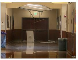
A broken ceiling piece hanging above a hallway after a 2,500 square foot section of roof at Capital High School in Olympia, WA collapsed in 2008. Olympia Assistant Fire Chief Greg Wright said the roof appears to have caved in due to the weight of snow, ice and water on top of the building. *(AP Photo/The Olympian, Steve Bloom)*
