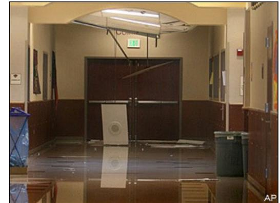
A broken ceiling piece hanging above a hallway after a 2,500 square foot section of roof at Capital High School in Olympia, WA collapsed in 2008. Olympia Assistant Fire Chief Greg Wright said the roof appears to have caved in due to the weight of snow, ice and water on top of the building. *(AP Photo/The Olympian, Steve Bloom)*
